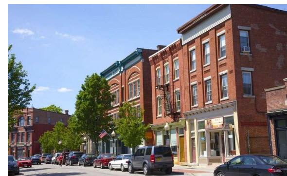
3-story MXU multifamily
