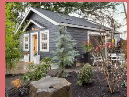
Detached garage conversion
