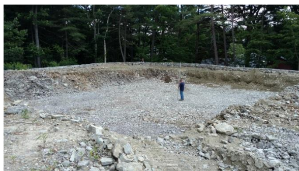
Finish Grading for Lot 6 Foundation (6/21)
