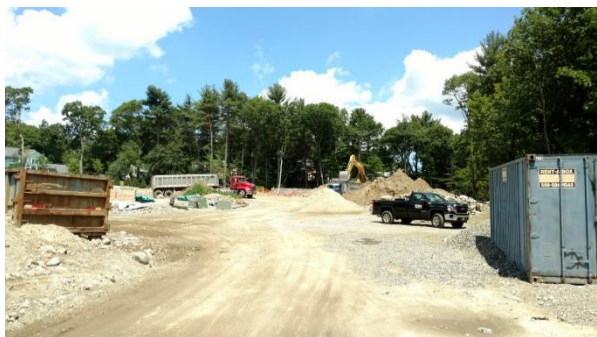
Stockpile Removal from Lot 7 (6/21)
