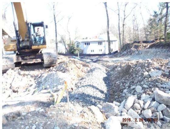
Infiltration unit Lot 1 connected to infiltration unit
