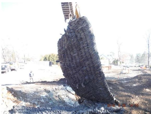
Blasting mats being set in place prior to first blast
