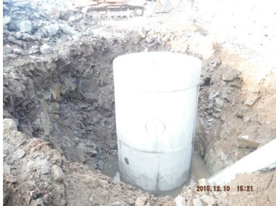
Titan sets DCB 3 rear lot 3 in proposed swale 12/10/15
