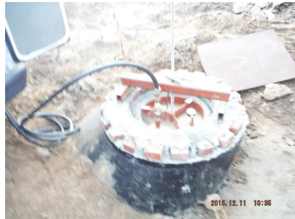
Sewer manhole vacuum testing completed 12/11/15
