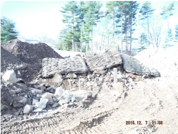
Blasting 12/7/15 on hold until further notice
