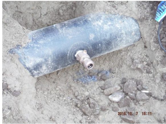
Corporations for house services installed 12/7/15
