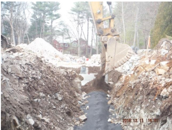
8" perforated underdrain pipe connected CB 3 to CB 2 12/11/15
