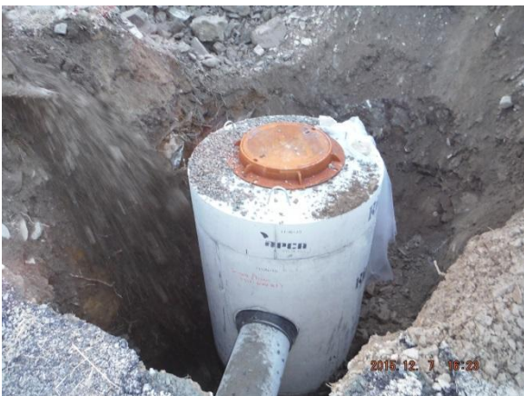
Water Quality Unit installed STA 1+35 12/7/15
