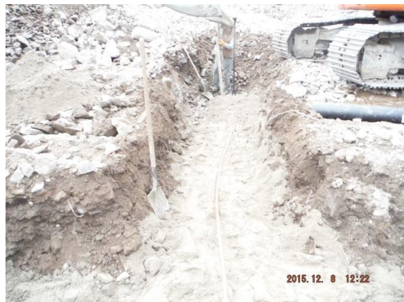
Water services and shutoff installed to all house Lots 12/8/15
