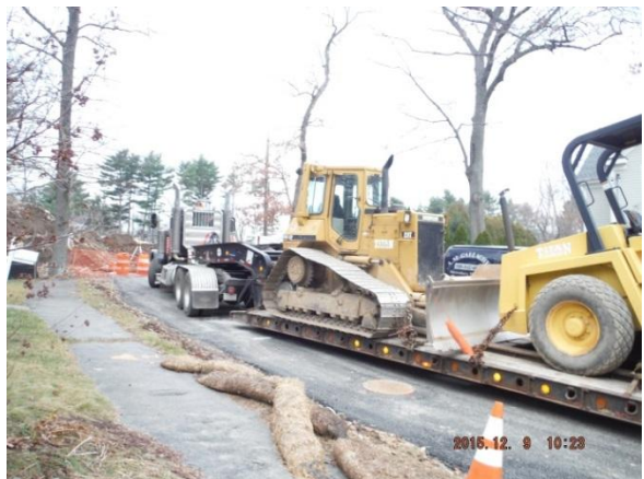
Titan delivers bulldozer & vibratory roller 12/9/15
