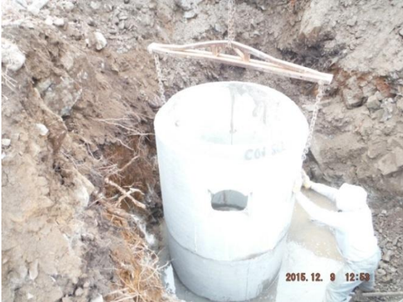
Catch Basin 1 installed STA 1+40 - 12/9/15
