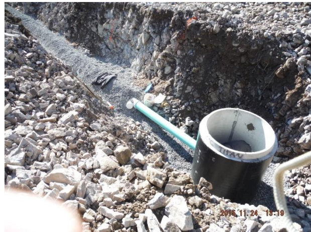
Titan installs Sewer Manhole 6 STA 5+46 11/24/15
