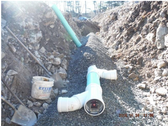
Installation of sewer wyes for individual lots 11/24/15
