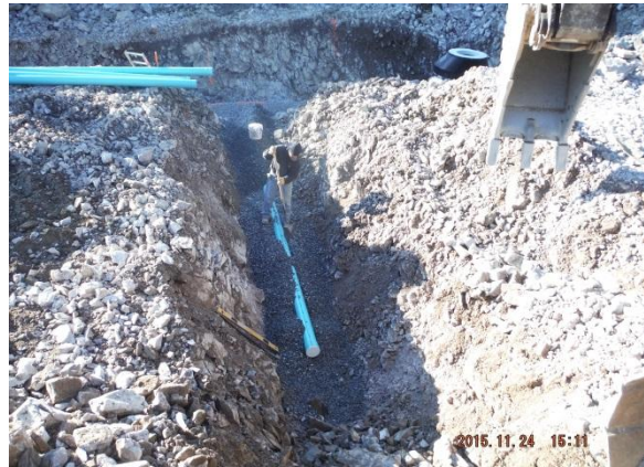
Installation of sewer lateral Lot 7 11/24/15
