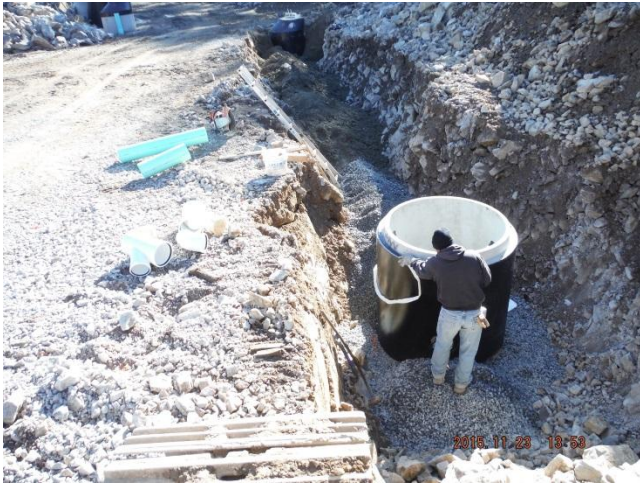
Titan installs Sewer Manhole 5 STA 4+12 11/23/15
