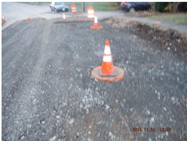
Rockwood Lane prepared for paving 11/24/15
