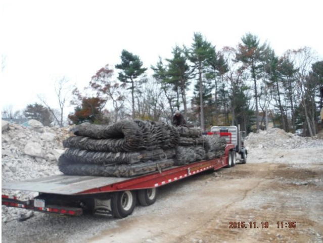
Blasting mats loaded and hauled offsite 11/19/15
