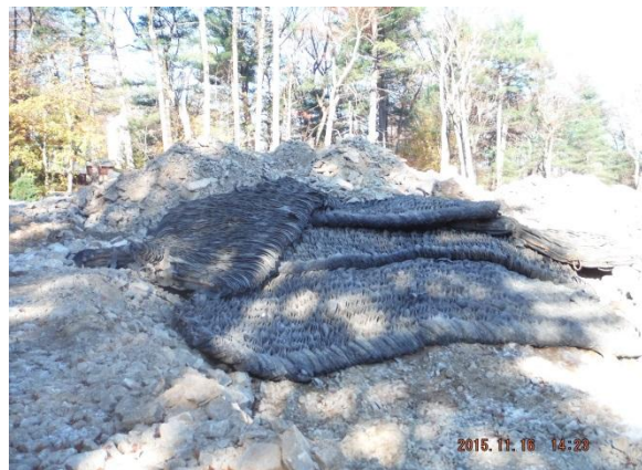
Blasting mats set for first blast Lot 4 11/16/15
