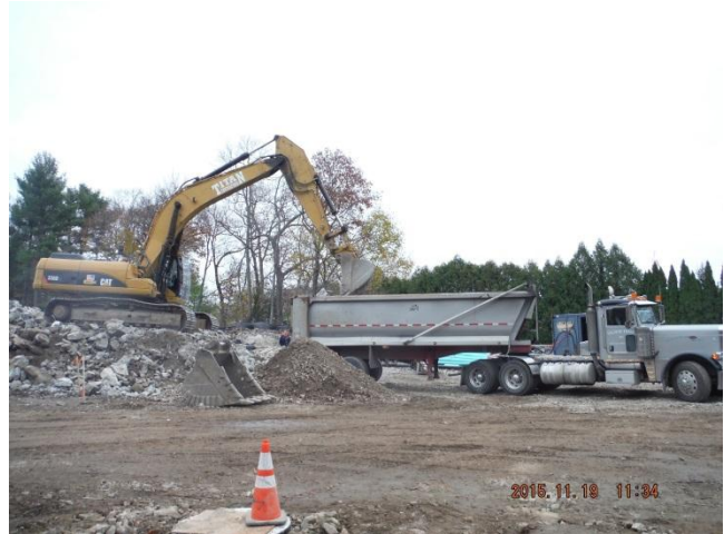
Blasted rock loaded and hauled offsite 11/19/15
