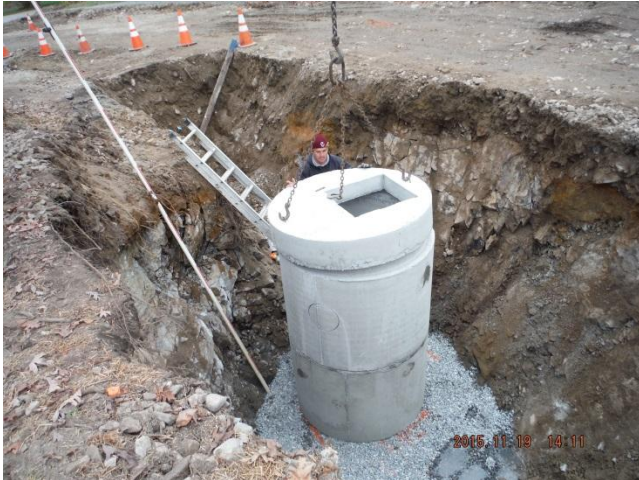
Set Catch Basin 2 STA 1+53 11/19/15
