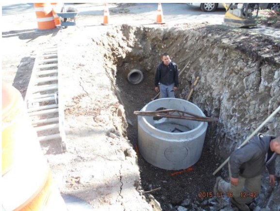
Set Drainage Manhole 1 STA 0+56 11/16/15
