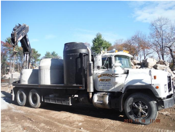
Delivery of Sewer & Drainage Manholes 11/17/15
