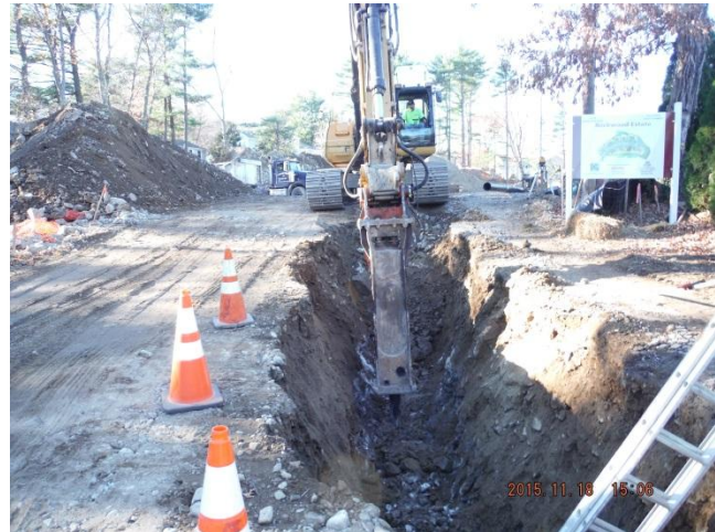
Titan Contractors hammer ledge to extend water main on Rockwood Lane 11/18/15
