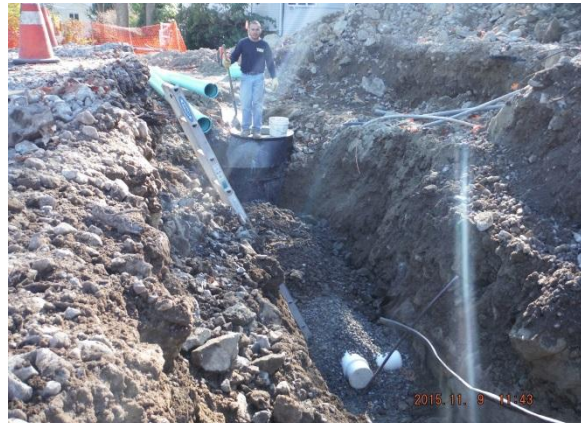
Sanitary Sewer connection for Lot 1 STA 1+82.5 11/9/15
