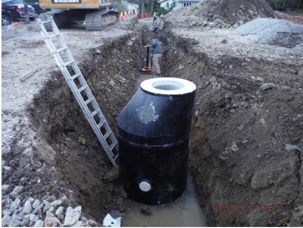
Sewer Manhole 3 STA 2+61 - 11/9/15
