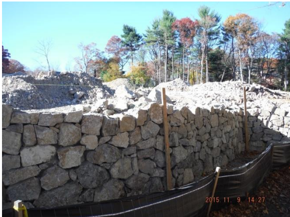
Retaining Wall behind Lots 7 & 8
