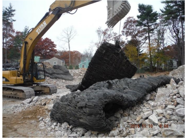
Setting Blasting Mats Lot 6 11/10/15
