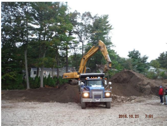
Hauling operations continue. Large stockpile completely screened 10/20/19
