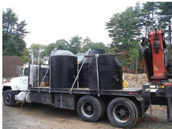
Sewer Man hole being delivered to the site 10/21/15
