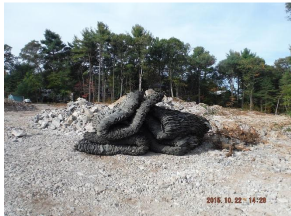
Blasting mats delivered to the site 10/21/15
