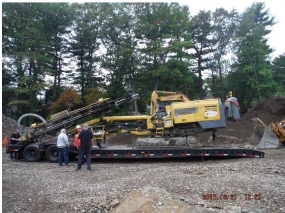
Drill rig being delivered to the site 10/21/15
