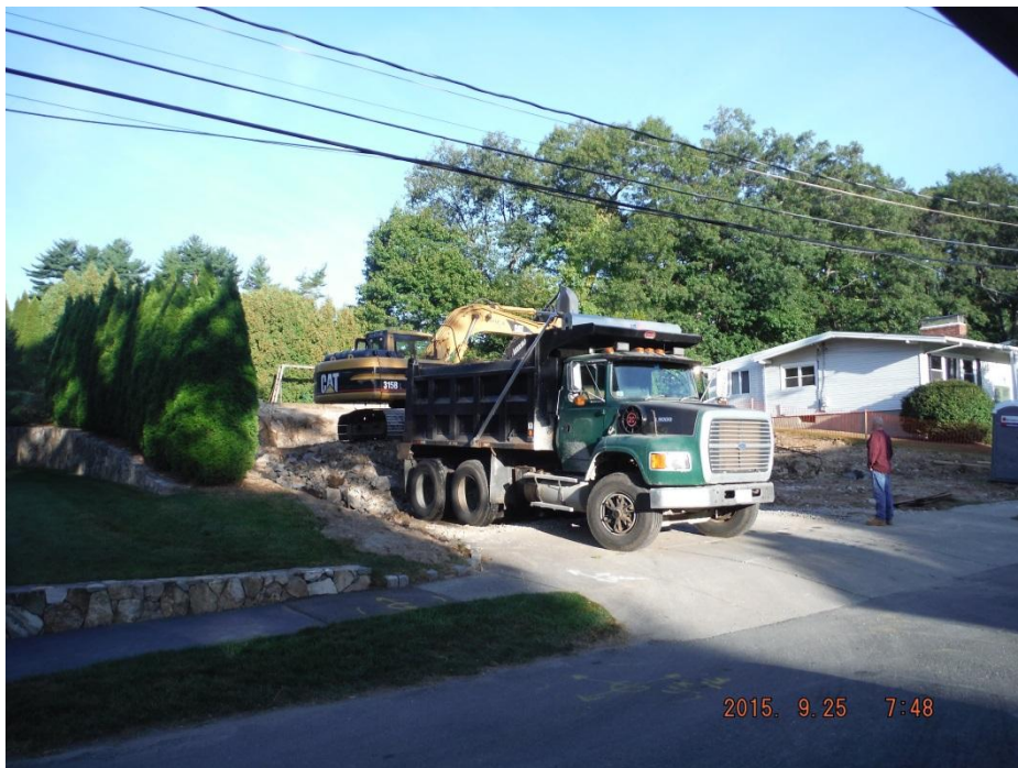
Ten Wheel truck hauling material from 79 Richard Road
