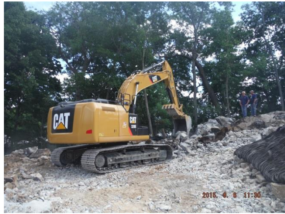
Excavation of blasted rock
