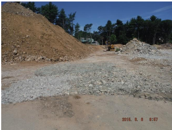
Construction pad installed 8/04/15
