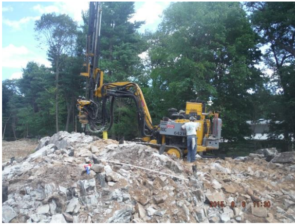
Rock Drilling Continues Daily
