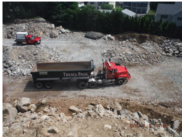
Trailers hauling excavated rock offsite
