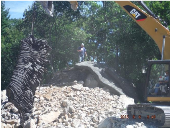
Setting blasting mats prior to blasting
