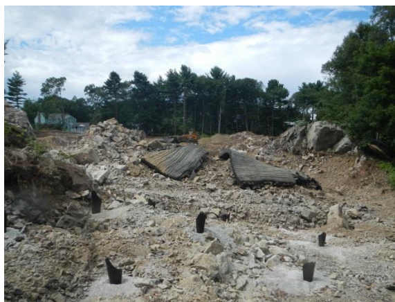
Southeast Area of Site After Third Blast and Mats Removed
