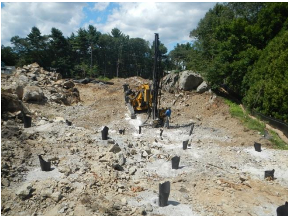
Rock Drilling Southeast Area of Site
