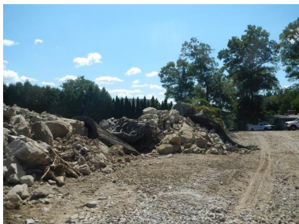
Ledge After First Blast and Mats Removed (Reverse Angle)
