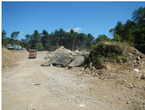
Site Prepared for First Blast
