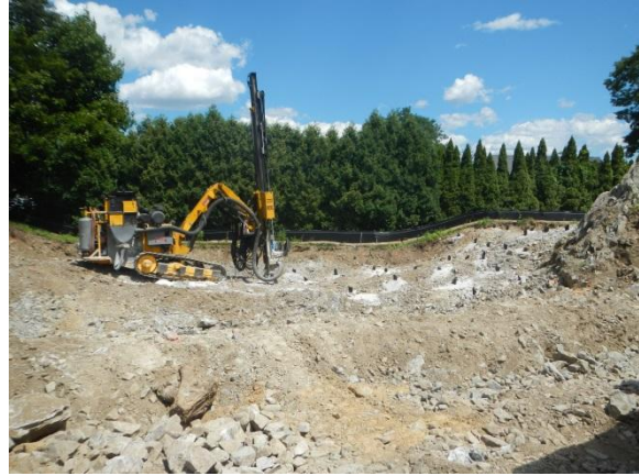
Rock Drilling Southeast Area of Site
