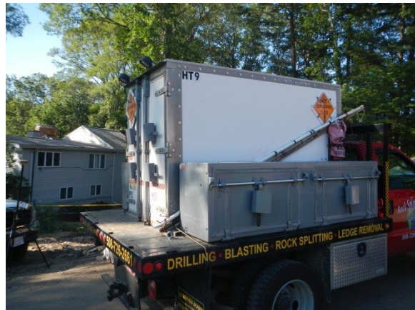
Explosives on Site (Removed at End of Workday)
