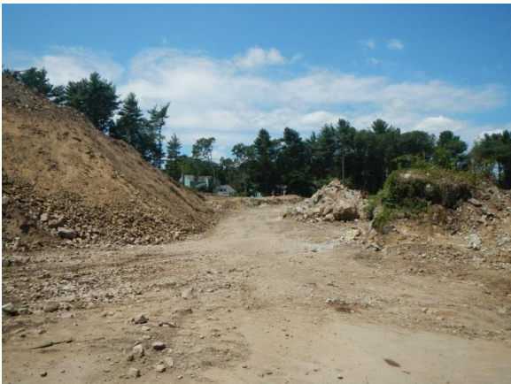
View from site entrance
