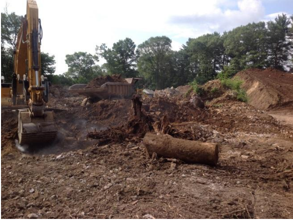
Excavation down to ledge
