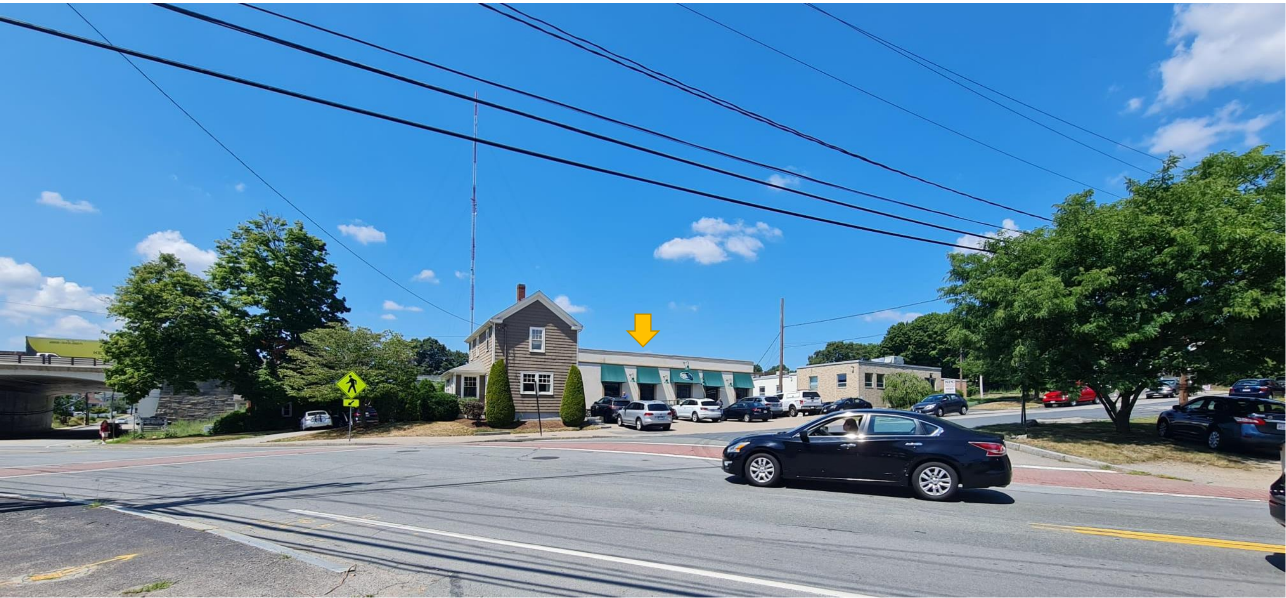
Fallon Custom Homes 171 Reservoir Street, Needham
