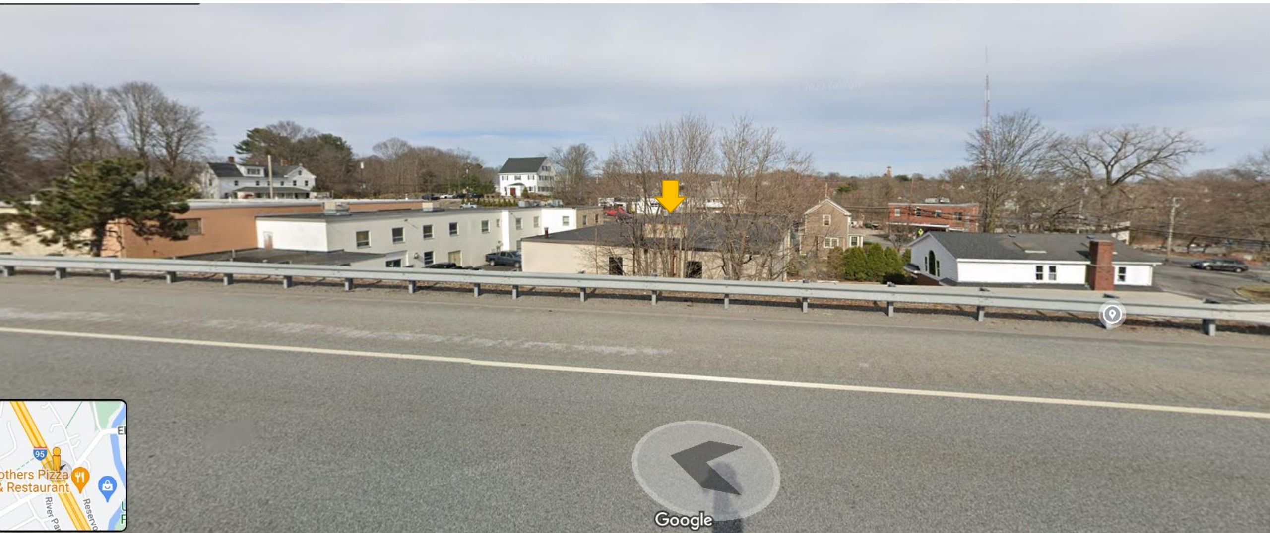
Fallon Custom Homes 171 Reservoir Street, Needham
