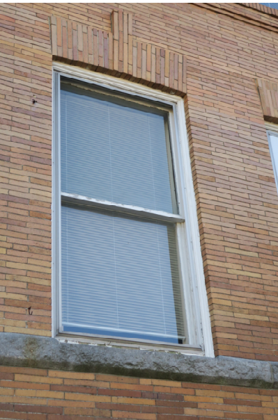
Existing painted wood windows with single glazing
