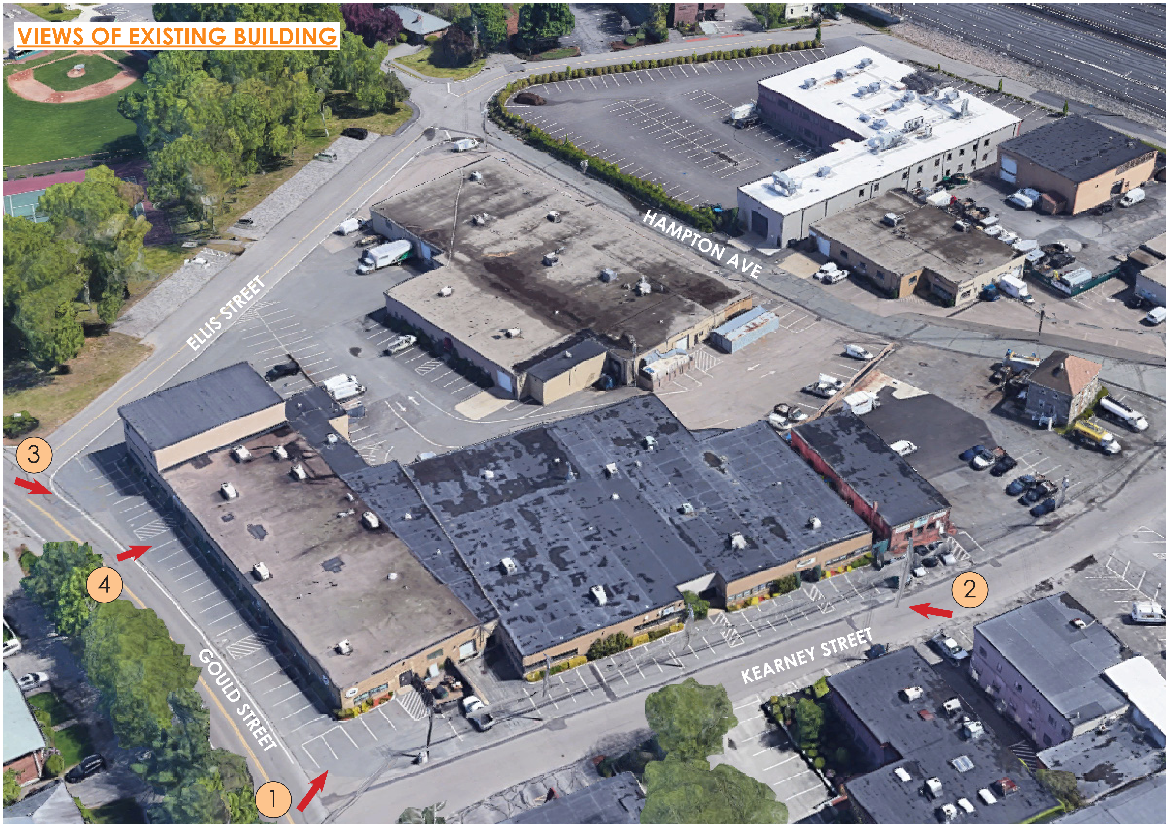
AERIAL SITE VIEW
