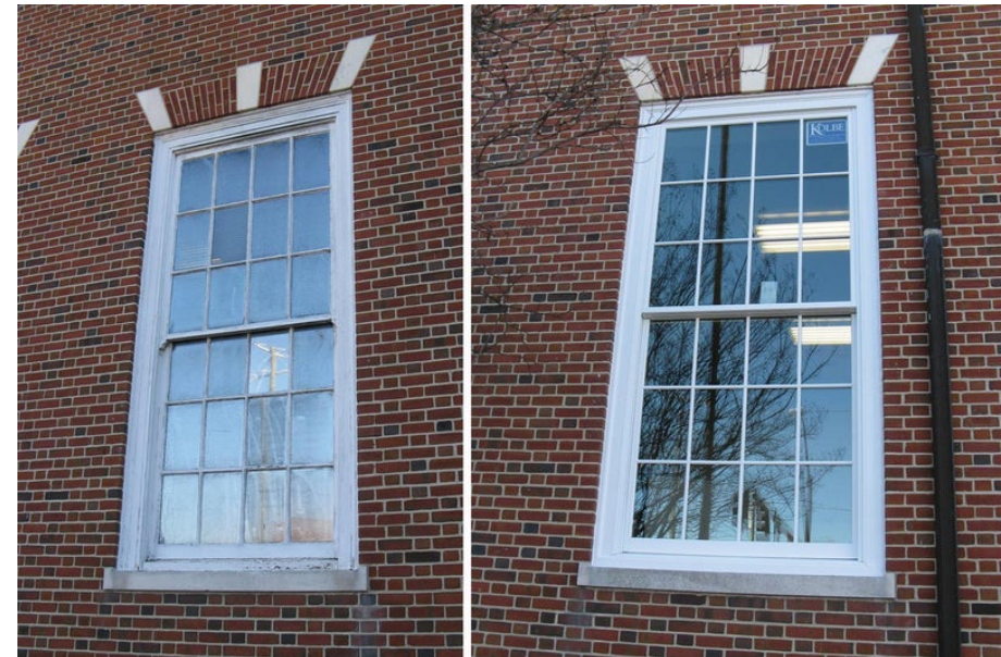
Example of aluminum clad wood with insulating glass
