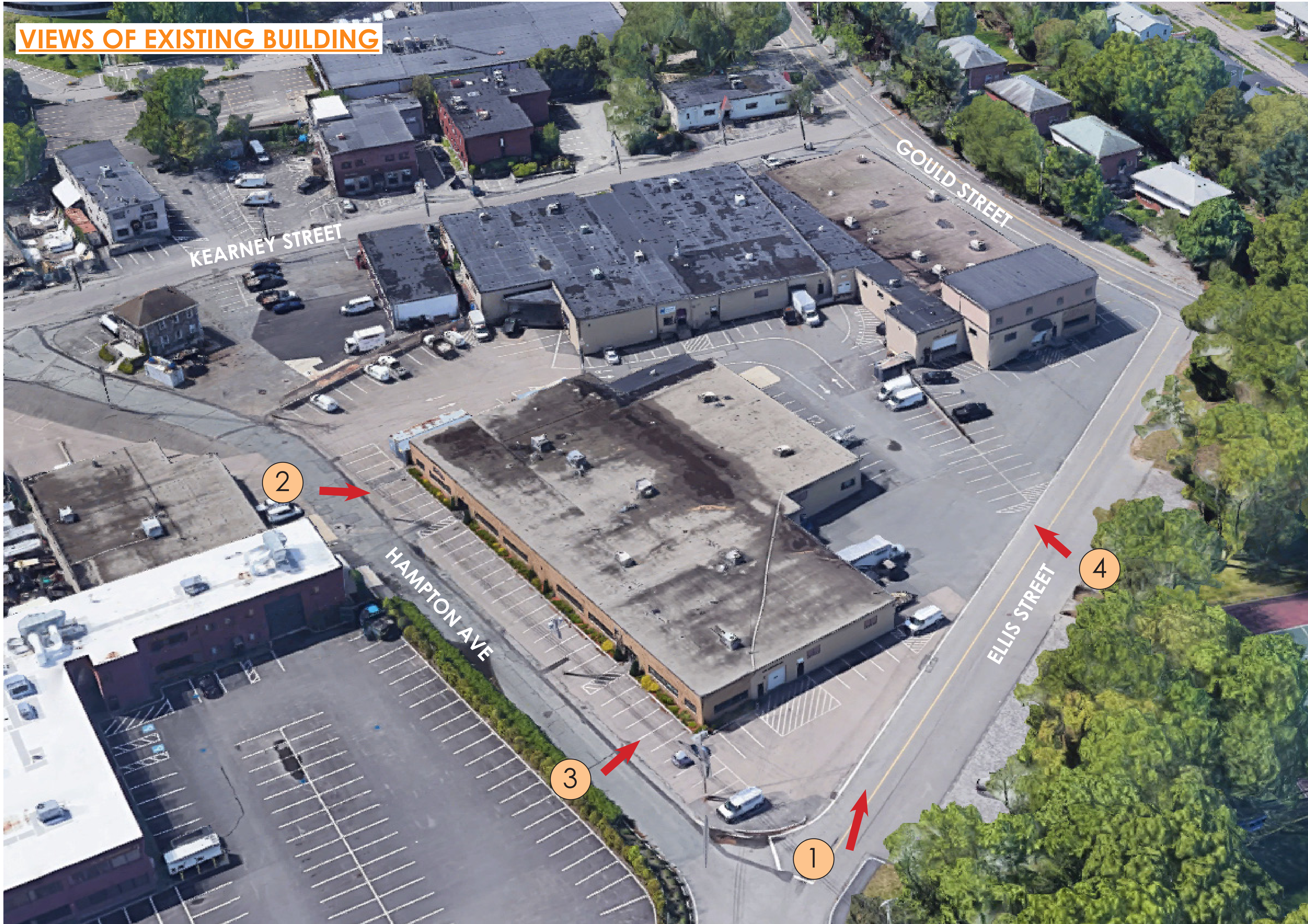
AERIAL SITE VIEW
