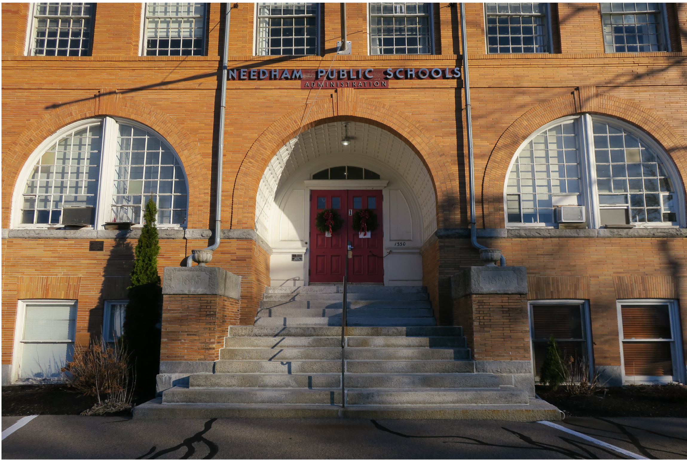
3 Existing Center Entry
