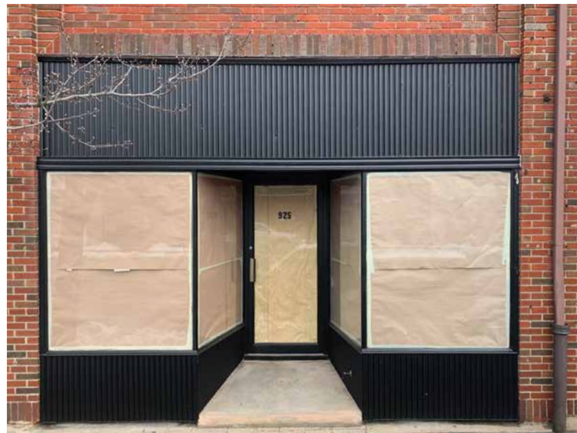
Current Facade (No Signage), After Refinishing
