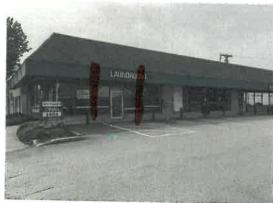
#3 CURRENT STOREFRONT FACING PARKING LOT
