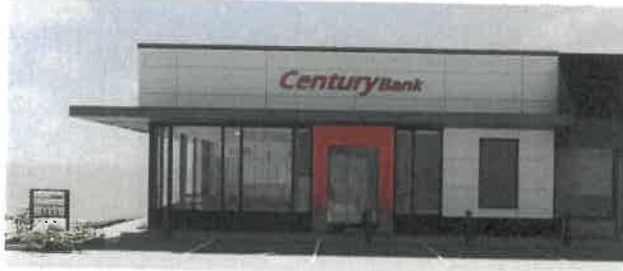
NORTH FACADE - PARKING LOT
