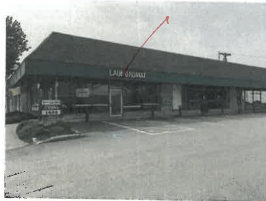
#3 CURRENT STOREFRONT FACING PARKING LOT
