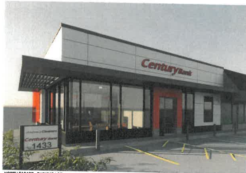
NORTH FACADE - PARKING LOT
