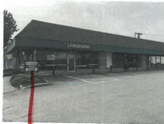
#3 CURRENT STOREFRONT FACING PARKING LOT
