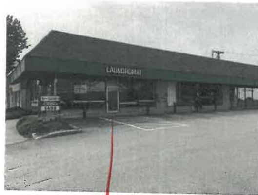
#3 CURRENT STOREFRONT FACING PARKING LOT
