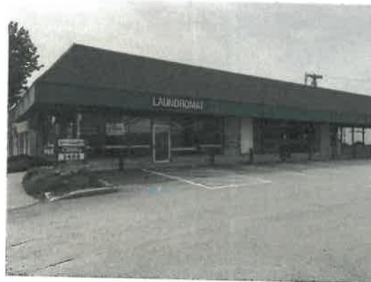
#3 CURRENT STOREFRONT FACING PARKING LOT
