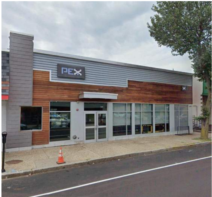
View C - North (Highland Ave side)
