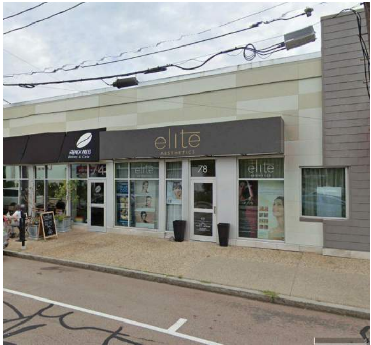
View A - North (Chapel Street side)
