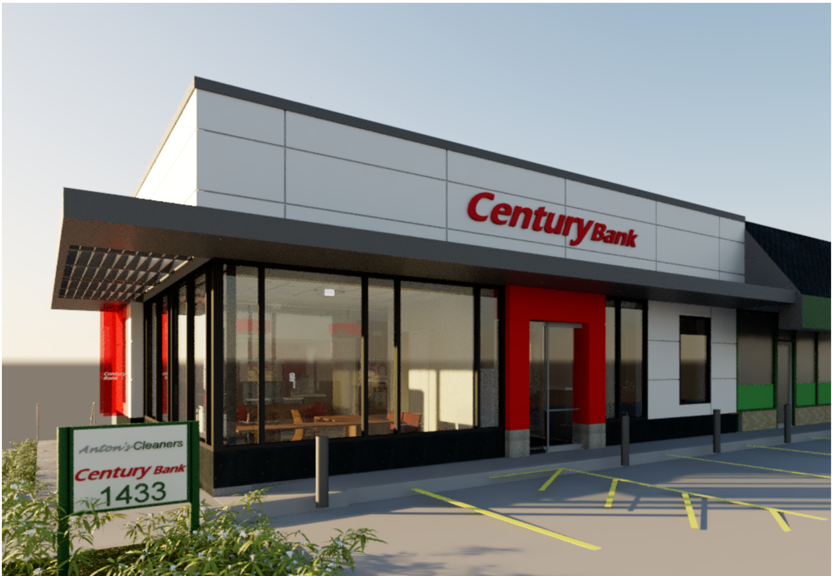
NORTH FACADE - PARKING LOT
