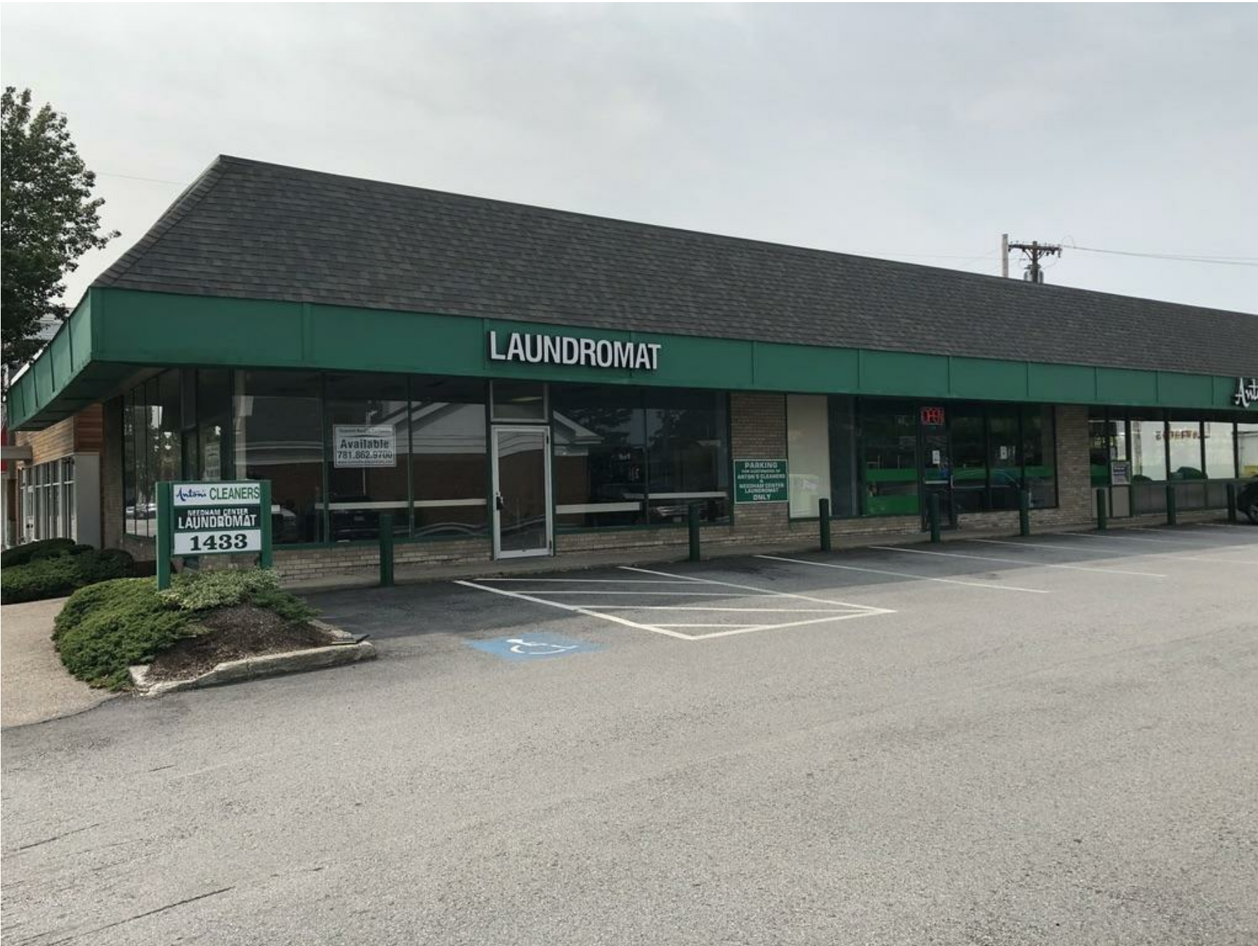
#3 CURRENT STOREFRONT FACING PARKING LOT
