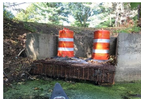
Outlet of Walker Pond on August 31, 2017. The water level was approximately 4 inches below the height of the spillway boards.
