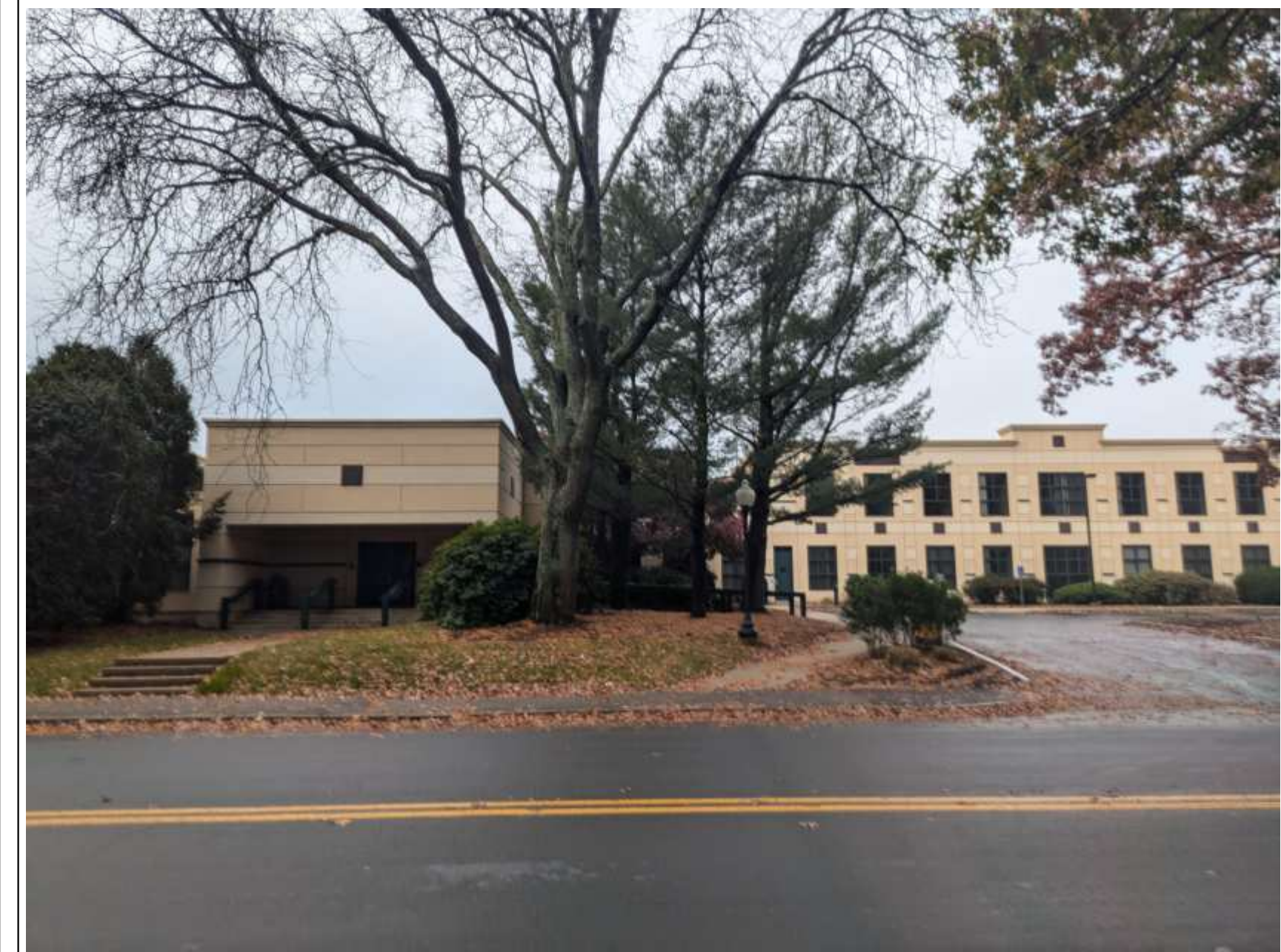
D: EAST FACE OF THE BUILDING FROM 4TH AVENUE
