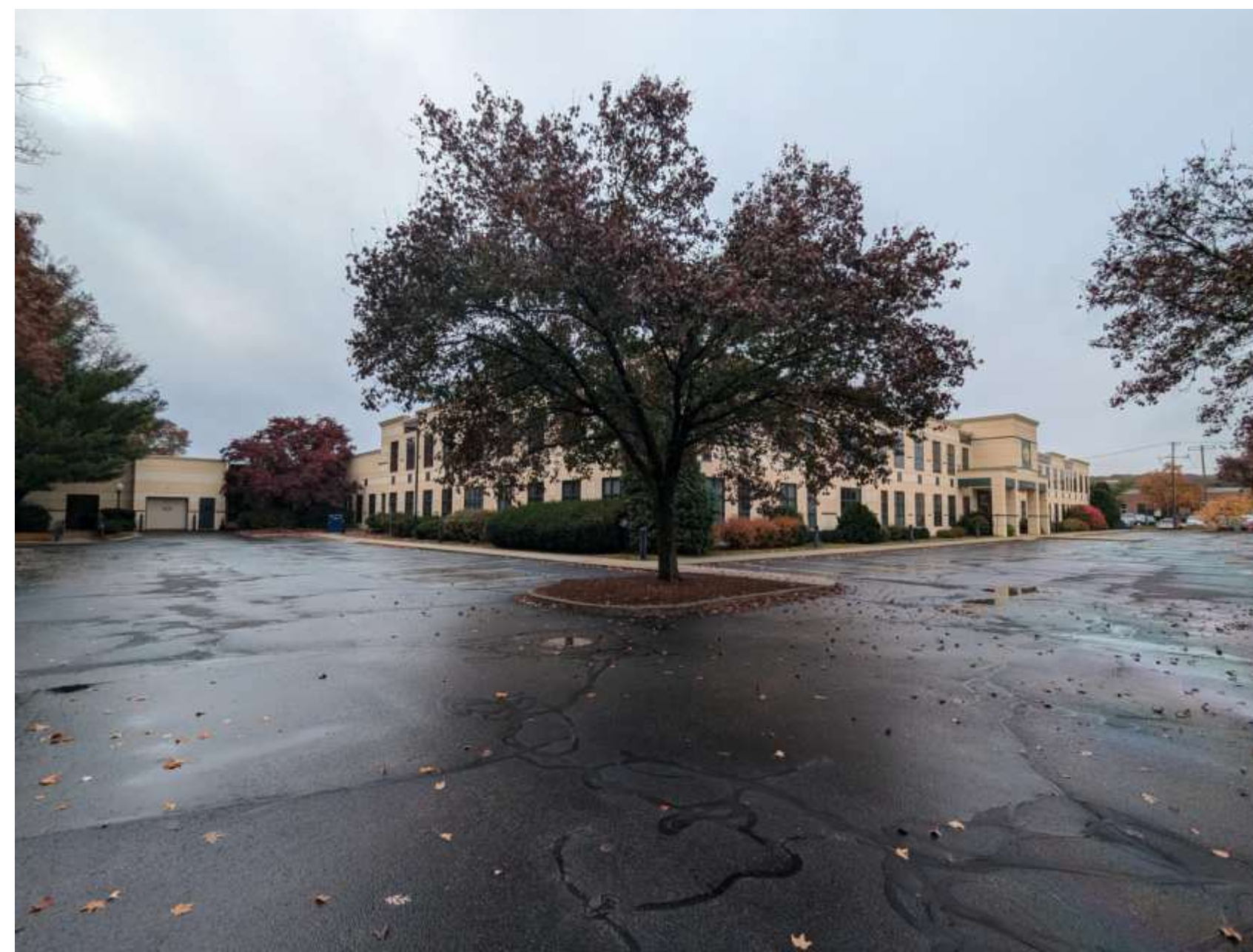
E: NORTH AND EAST FACE FROM REAR PARKING
