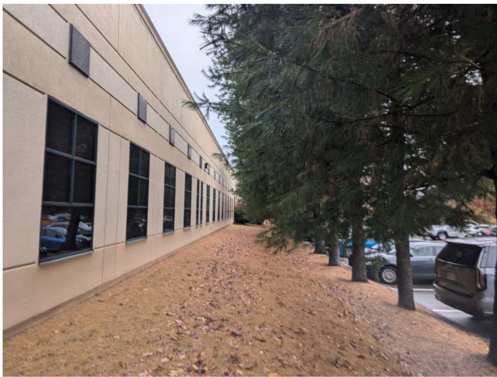
F: WEST FACE OF THE BUILDING
