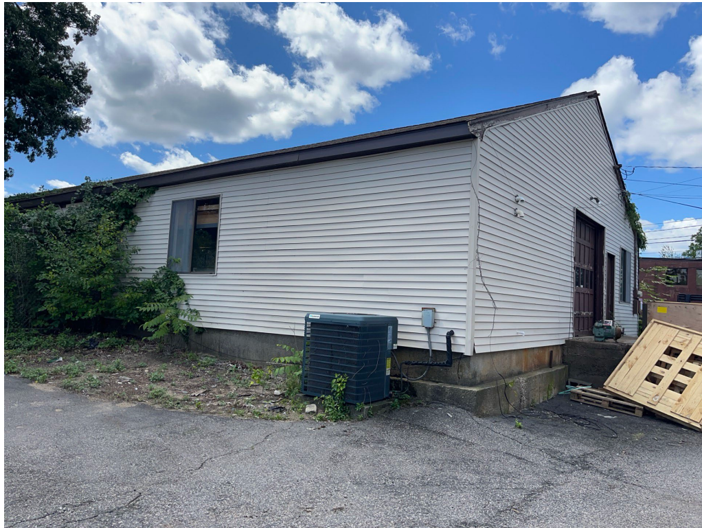
EXISTING: Northeast corner
