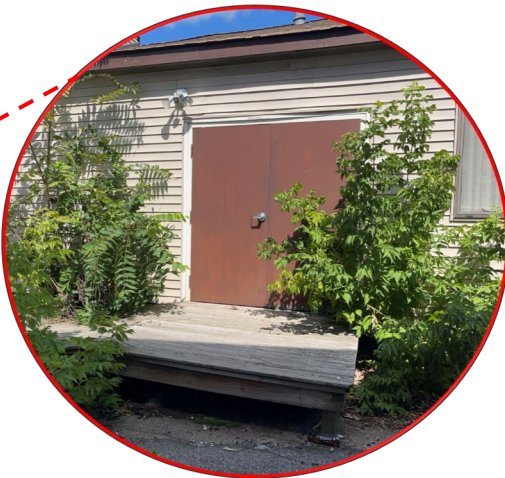
EXISTING: South deck & doors
