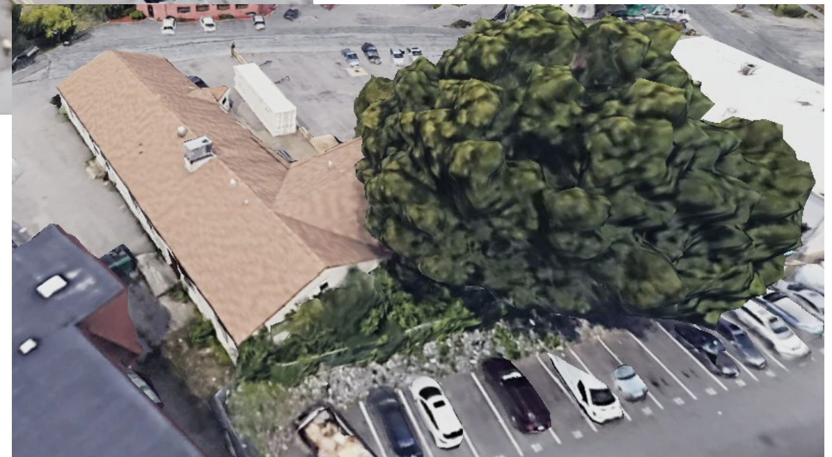
#2 EXISTING: Aerial of over-grown inaccessible Southeast corner and East elevation
