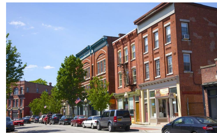
3-story MXU multifamily
