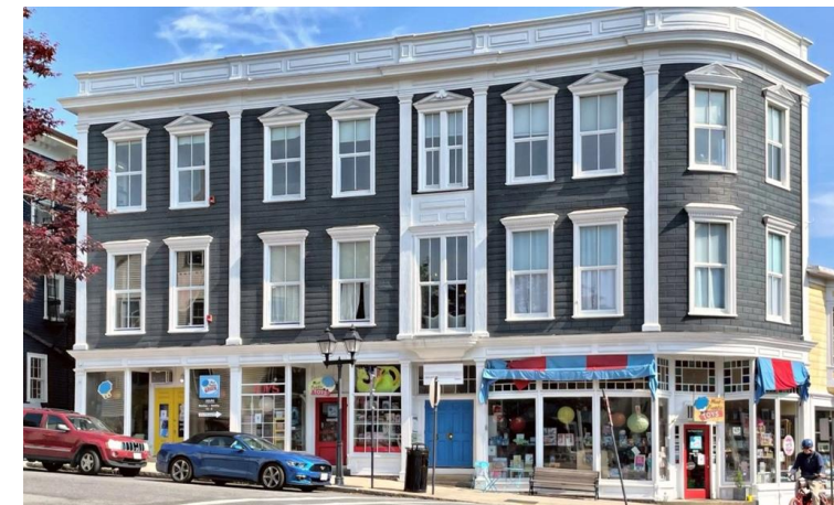
3-story MXU multifamily
