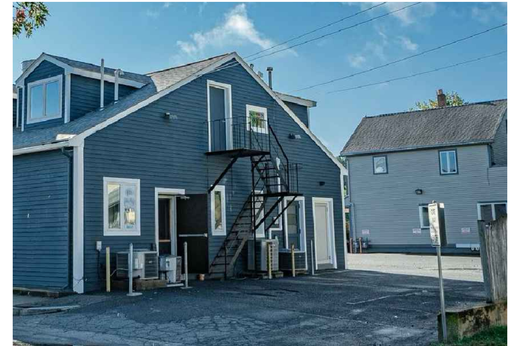
EXISTING REAR FACADE
