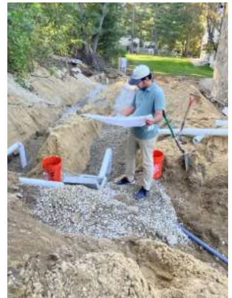
Sainath Palani, Environmental Health Agent, Conducting a residential septic system installation inspection.
