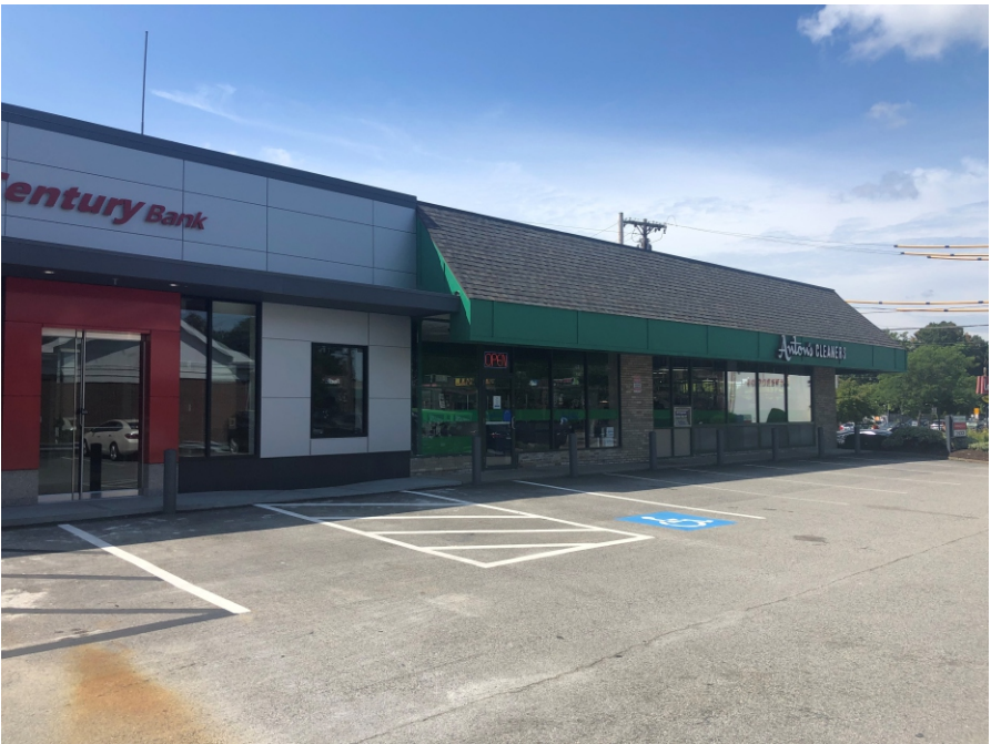
Front Elevation - Existing - Parking Lot View
