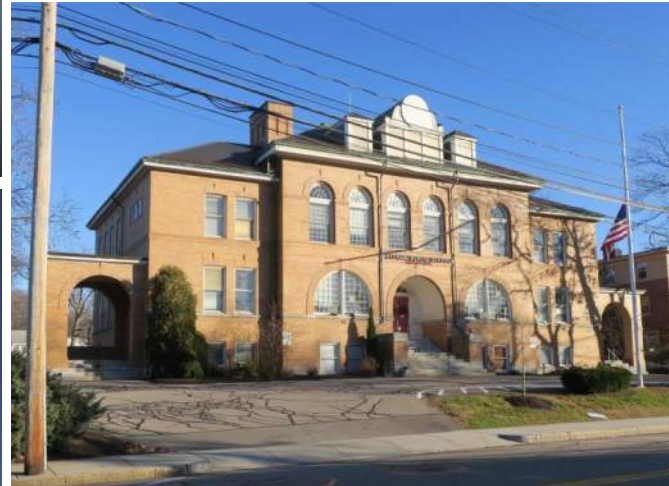
Emery Grover Renovations for School Administration Dept.
