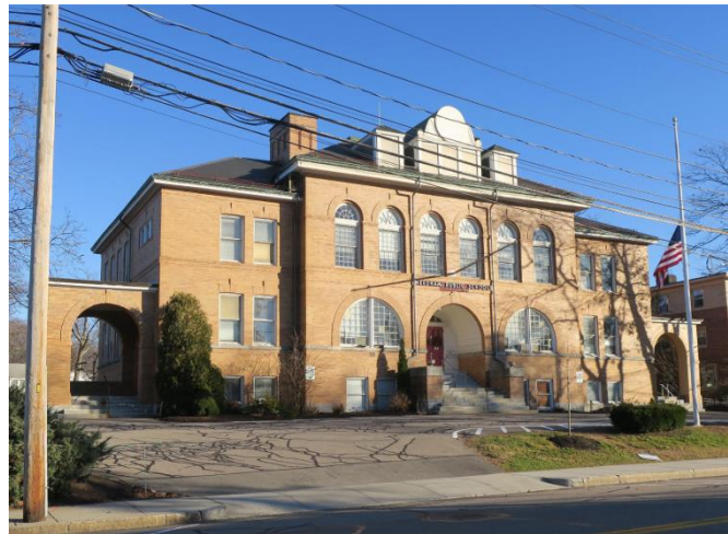
Emery Grover Renovations for School Administration Dept.
