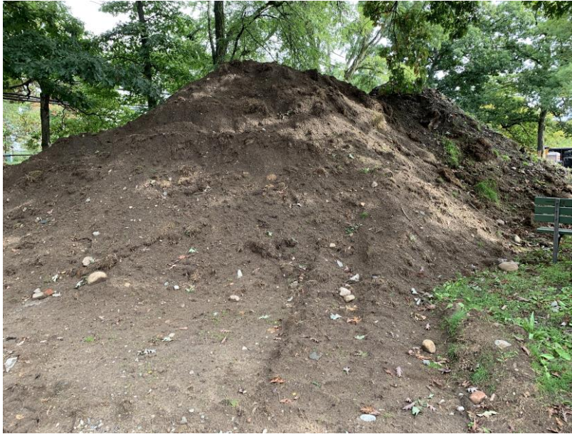
Photo 1. Stockpiled topsoil from laydown area.
