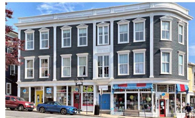
3-story MXU multifamily
