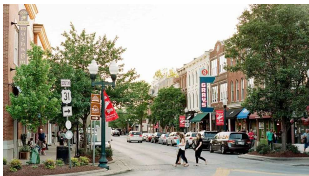
3-story MXU multifamily
