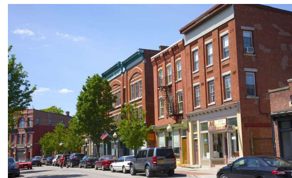
3-story MXU multifamily
