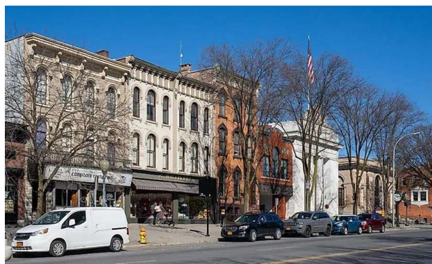
2-3 story MXU multifamily
