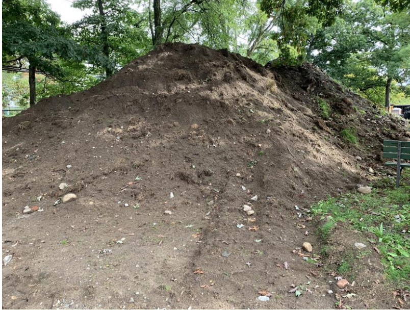
Photo 1. Stockpiled topsoil from laydown area.
