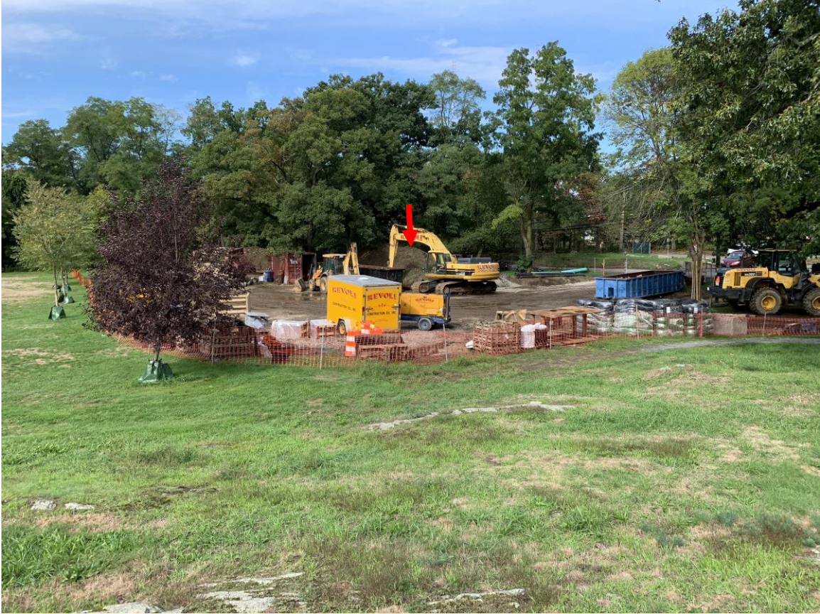
Photo 3. Laydown area overview, stockpile indicated by red arrow.
