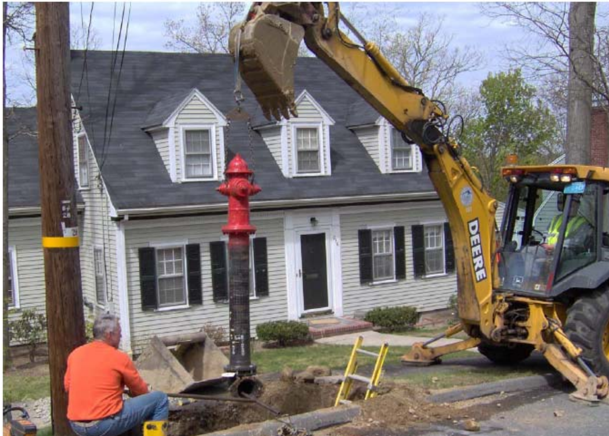
Fire Hydrant Replacement
