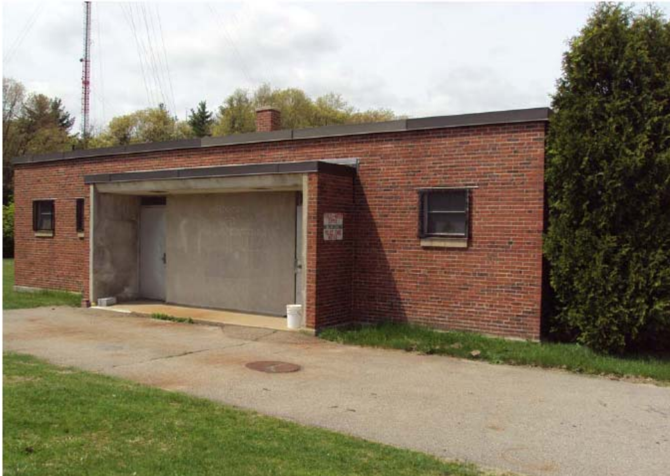
St. Mary Street Water Pump Station
