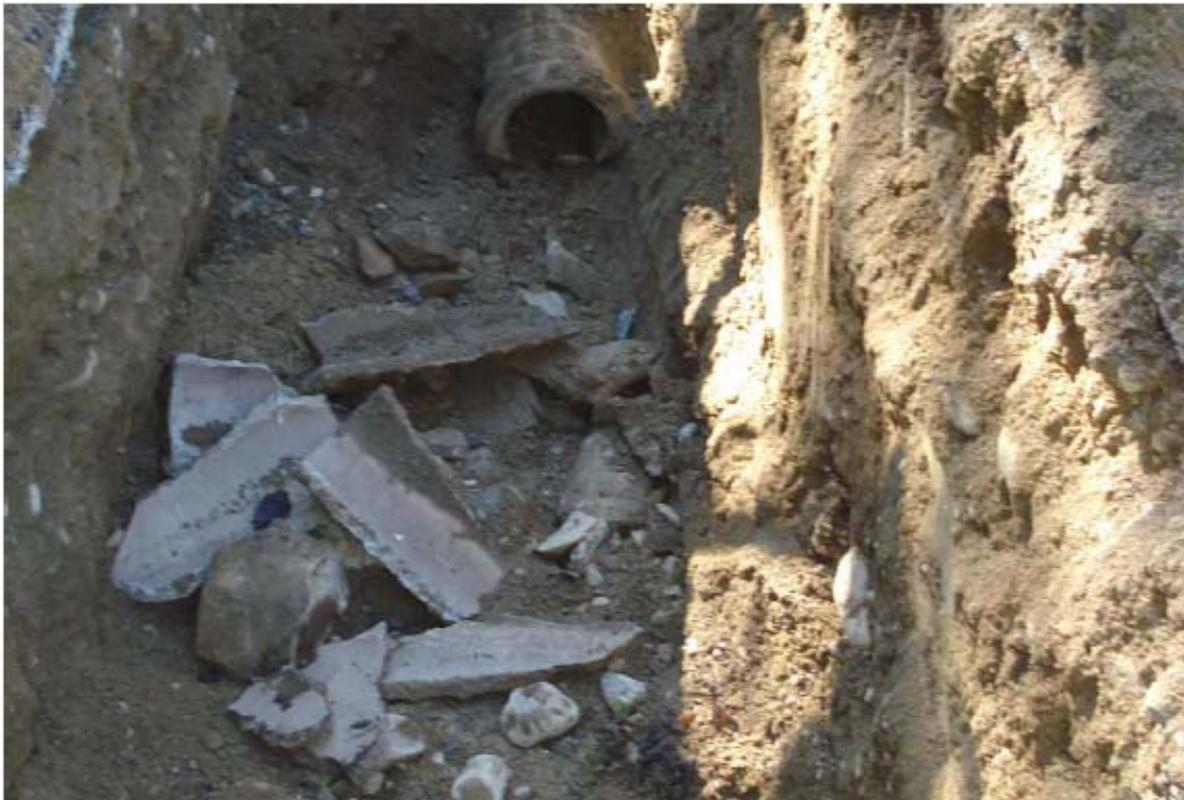
**Example of brittle sewer main that was a source of infiltration into the sewer system**
