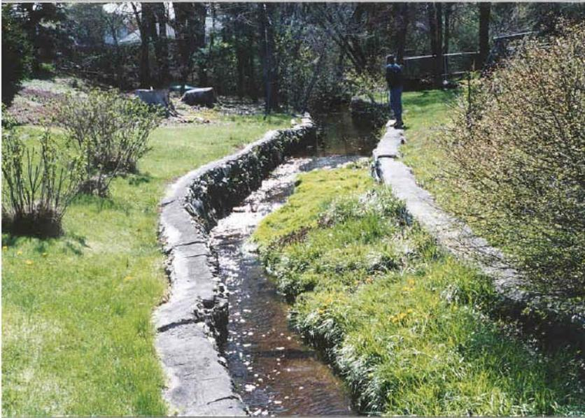
**Example of sedimentation into the stream channel, vegetation overgrowth and deteriorating channel walls.**
