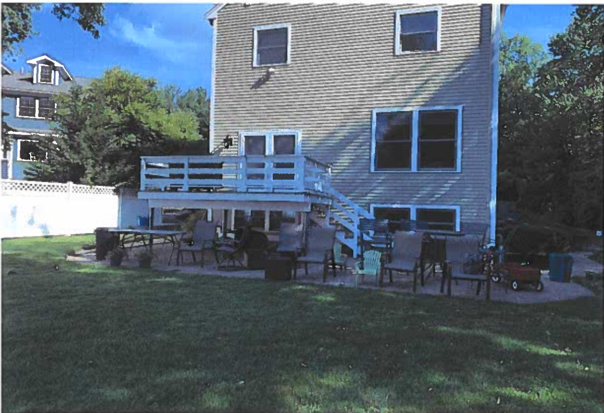
Existing patio and deck
