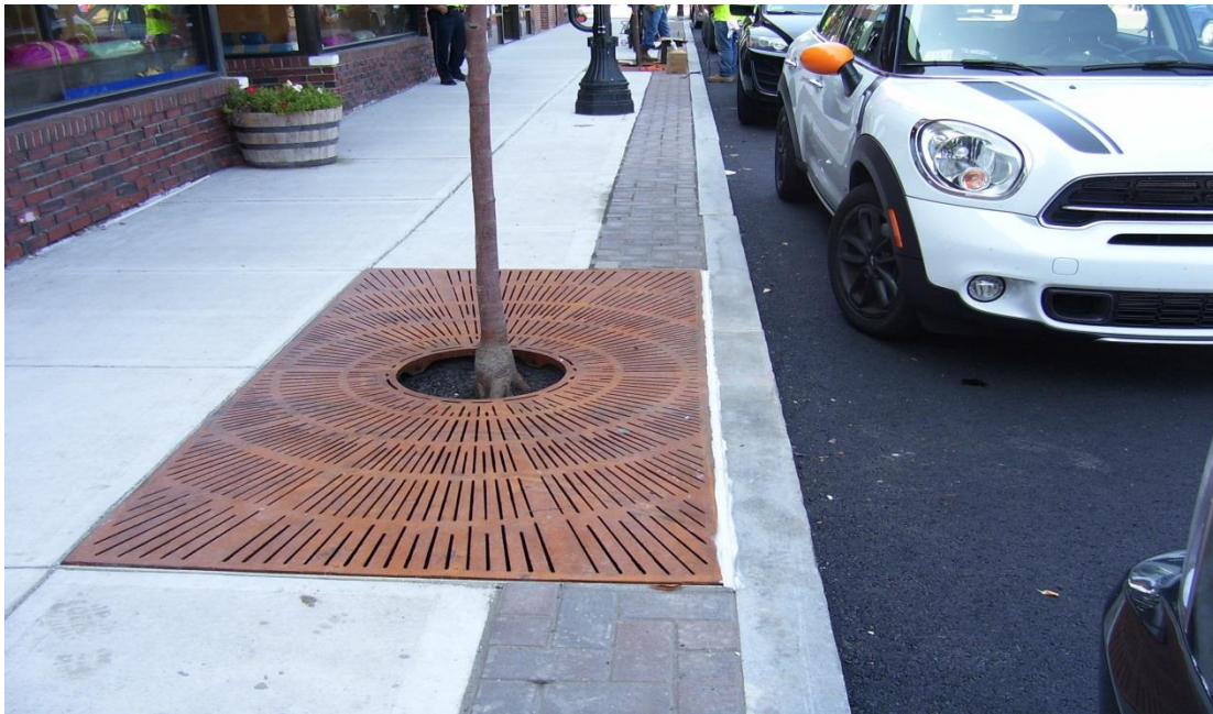
Caulking around tree grate
