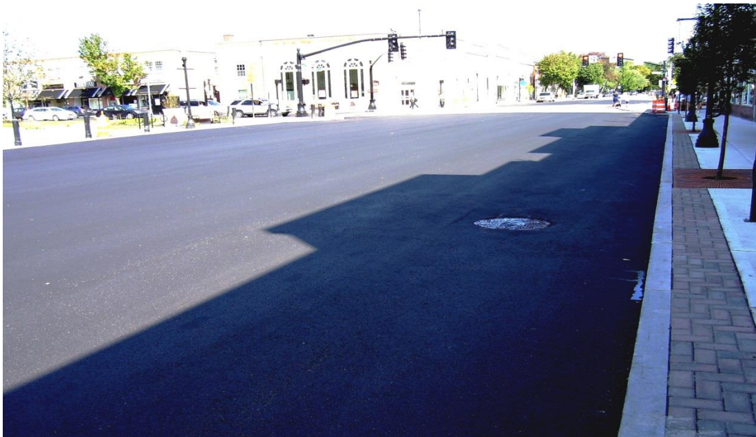
New paving looking northeast in Great Plain Ave. toward Highland Ave.
