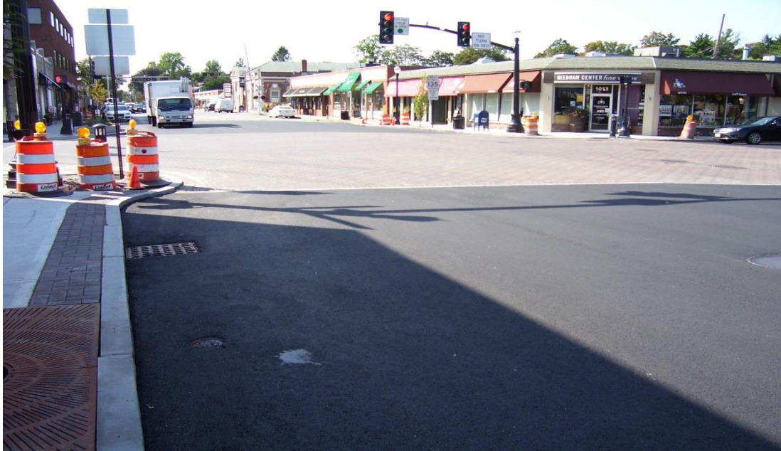
New paving looking northwest in Great Plain Ave. toward Chapel St.
