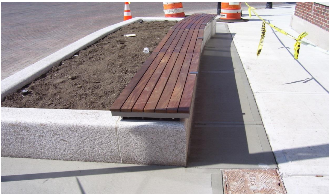
New granite planter with wood seat on the northeast corner of Great Plain Ave. and Highland Ave.
