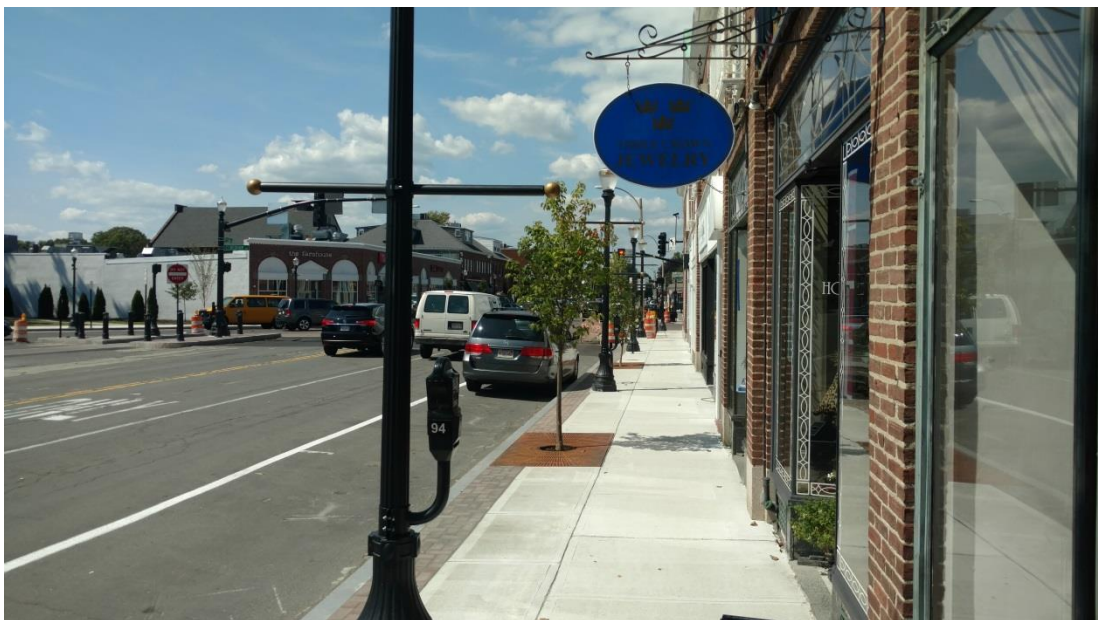
North side of Great Plain Ave. looking west showing typical sidewalk section
