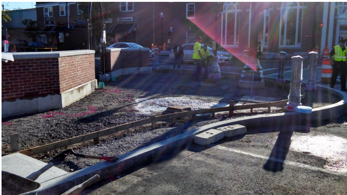
East side of the Common prepped for concrete walk and granite and brick paver base
