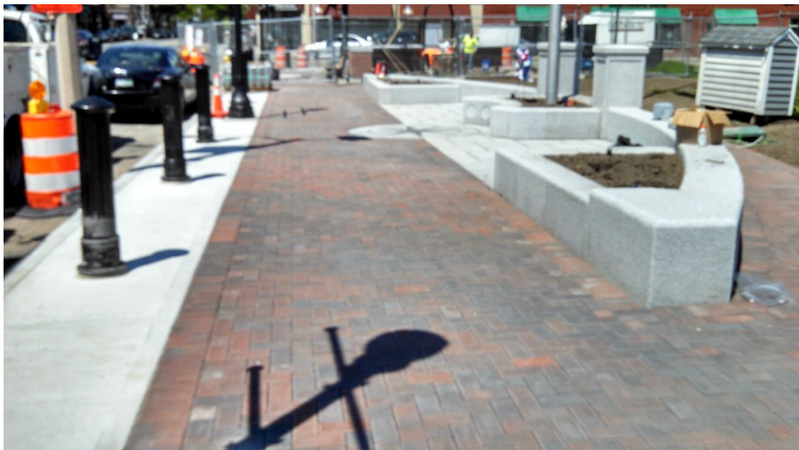
Brick pavers installed in front of the Common looking west
