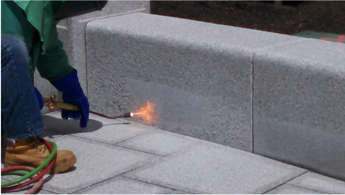
Thermal finishing of granite seat wall
