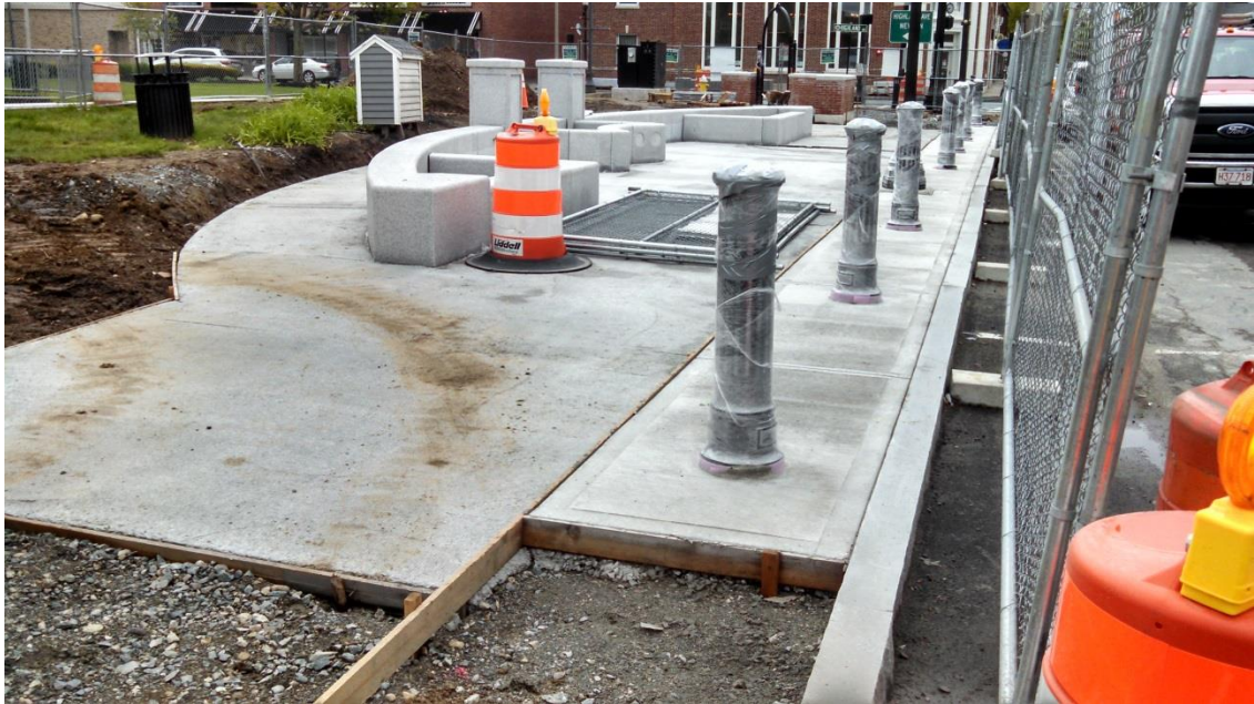
Concrete sidewalk and brick and granite paver base slab in front of Common looking east
