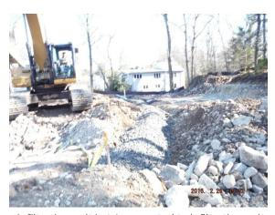
Infiltration unit Lot 1 connected to infiltration unit Lot 2 - 2/26/16
