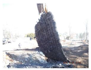
Blasting mats being set in place prior to first blast 2/26/16
