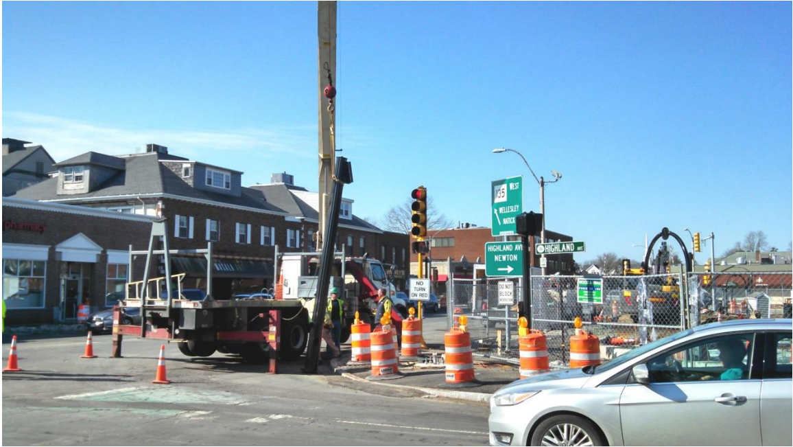
Setting mast arm pole on the northwest corner of Great Plain Ave. and Highland Ave.
