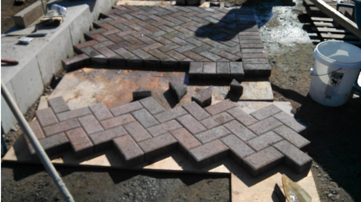
Mockup of brick pavers for Common and sidewalk areas
