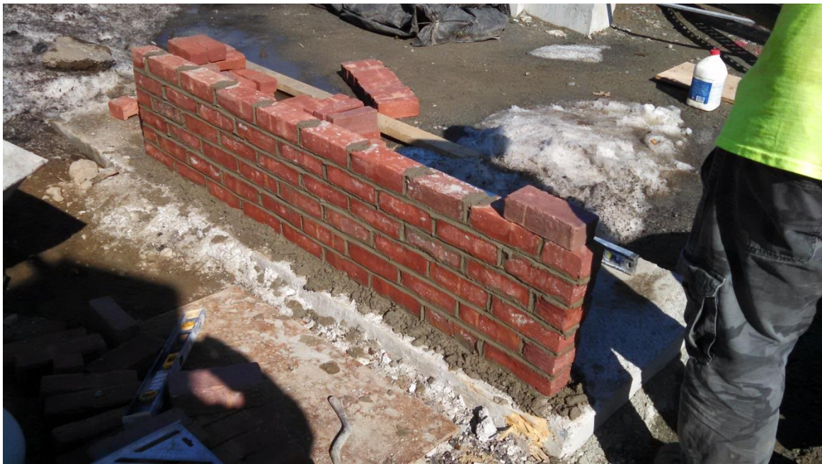
Mockup of brick wall for entrance to the Common
