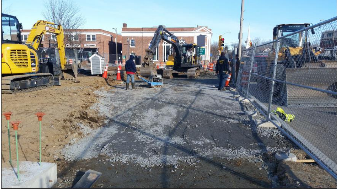
Installing and compacting gravel for brick paver base material
