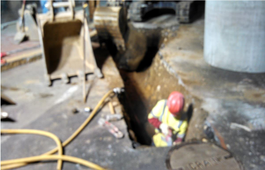
Installing drain lateral piping at station 10+68 in Great Plain Ave.
