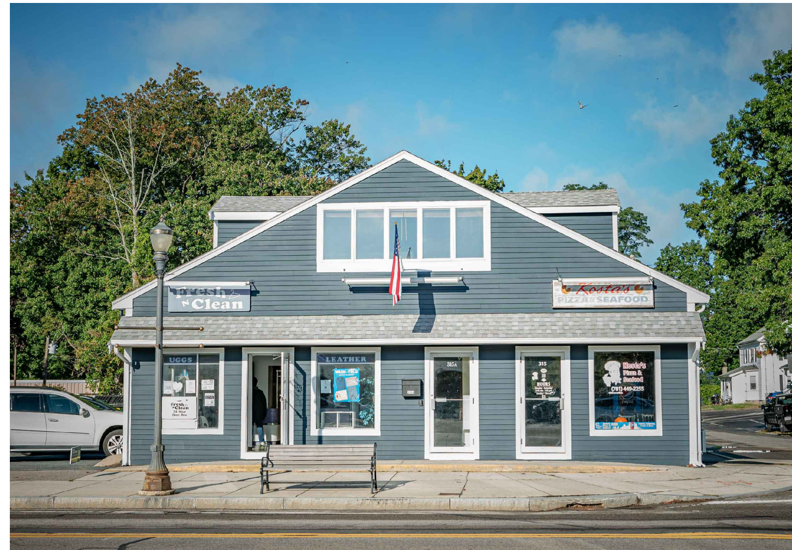
EXISTING FRONT FACADE CHESTNUT STREET
