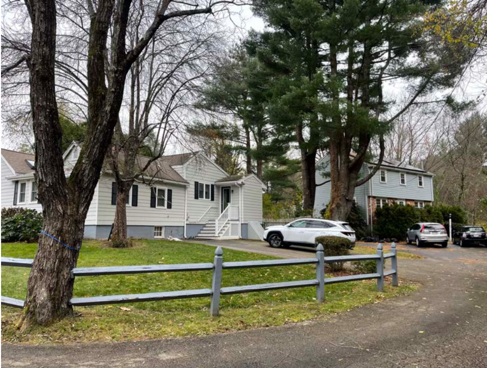
View of 20 Alder Brook Lane, showing driveway proposed to be removed
